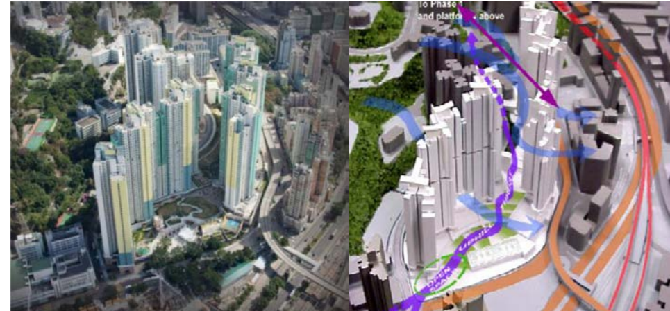
Fig. 2 (left) A bird’s eye view of the Upper Ngau Tau Kok Estate redevelopment project. (right) physical model with the design concept of introducing wind while fencing out traffic noise. Source: Hong Kong Housing Authority [17]s
