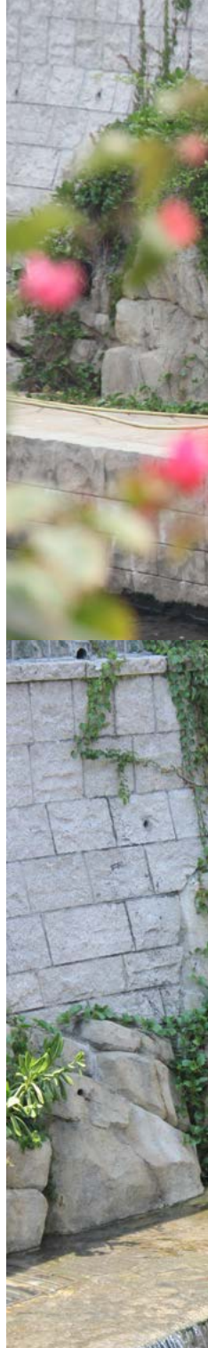
Fig.6 The artificial rock along the riverbed and riverbank is applied on an irregular basis to achieve a natural effect
