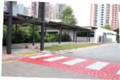
→ Strong colour contrast with the surroundings for greater visual clarity (applied where there is change in levels, as well as between walls, floors, furniture or fittings)
